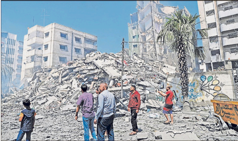
DESTROYED People inspect the rubble of the Yazegi residential building that was destroyed by an Israeli airstrike in Gaza City (AP Photo/Adel Hana).
